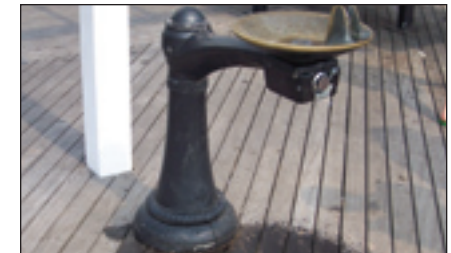
This Drinking Fountain's score was impacted by a steady leak. The fountain could not be turned off.
