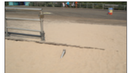
Entrances to the beach should be safe and clearly marked. This railing buried in sand is a hazard.
