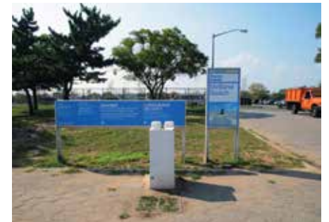
Midland Beach's concrete drinking fountains are in poor working condition
