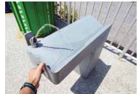
A drainless drinking fountain directs water and debris away from the user into a ground-level drain: it's usable even if the drain is clogged
