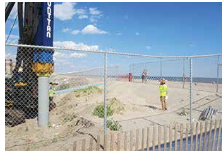
Construction at Rockaway Beach includes driving piles to support boardwalk reconstruction.
