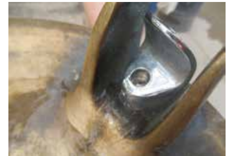
It is not possible to drink at this water fountain due to low water pressure
