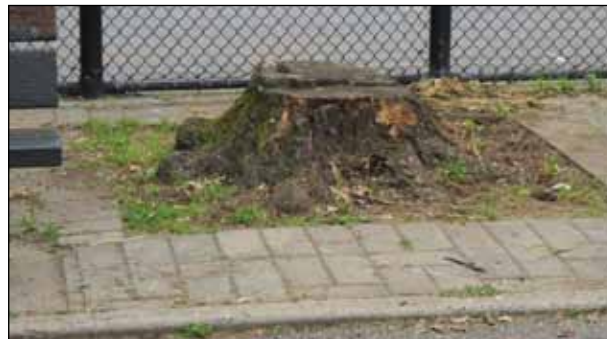
Tree pits with stumps and empty tree pits received failing grades.
