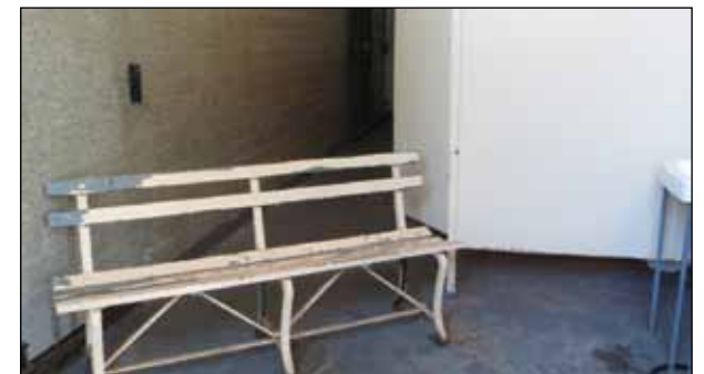
Surveyors encountered bathrooms that were used as storage areas.
